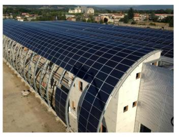
Tigo's panel-level MPPT corrects for mismatch caused by the curved façade and shade cast by nearby light poles.
